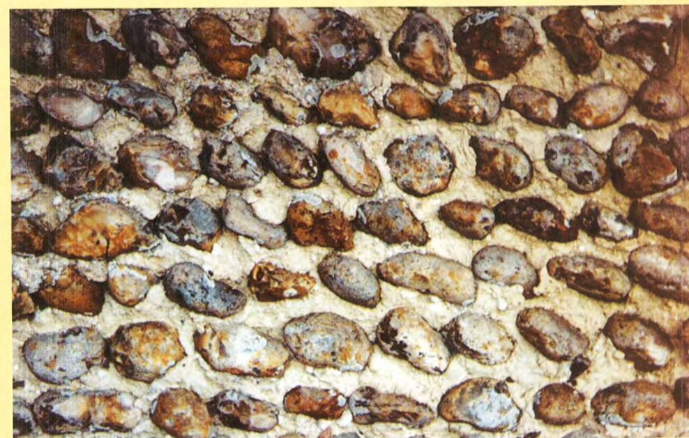
Original lime mortar still performing well after 200 years
